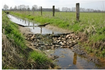
Damming of overflow
